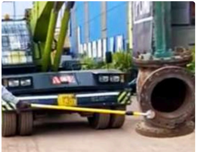
Crane-side pipe guidance — operator at defined working distance while crane supports the load
